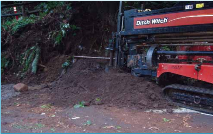
The horizontal drill rig inserting pipe along road
