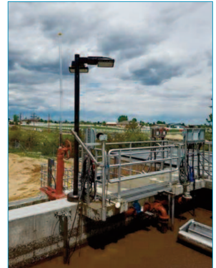
View From Top of New Concrete Tank
