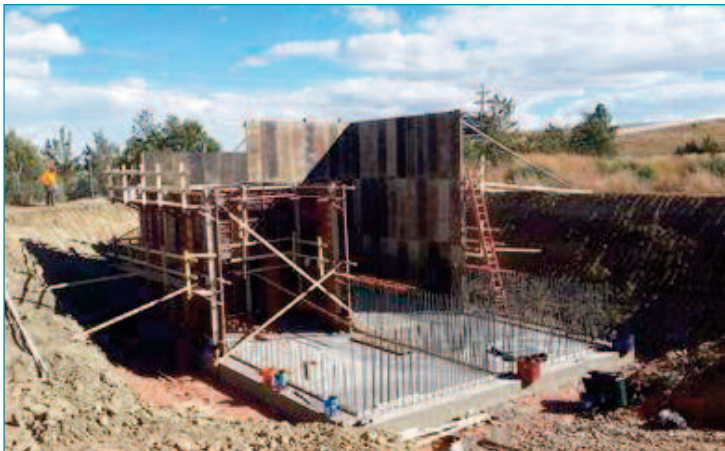
Forming Concrete Tank
