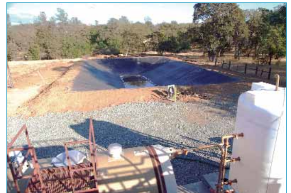
View of construction holding pond
