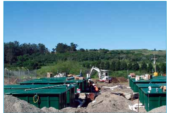
Advantex system under construction
