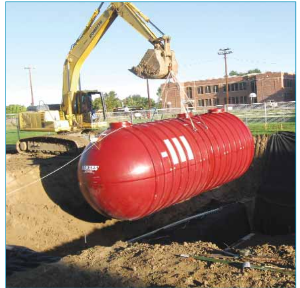
Setting the Xerxes Tank
