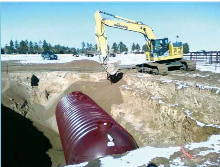
IWS installing fiberglass treatment tanks
