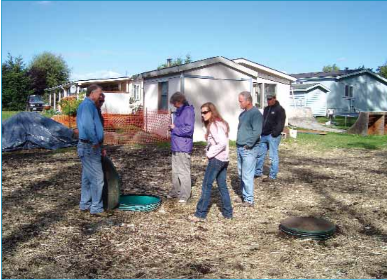
Project involved work in close proximity to homes
