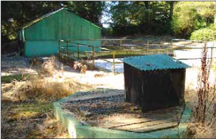
SSSD facility prior to upgrade
