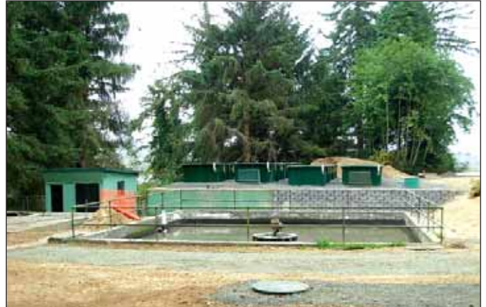
SSSD facility after upgrade was completed
