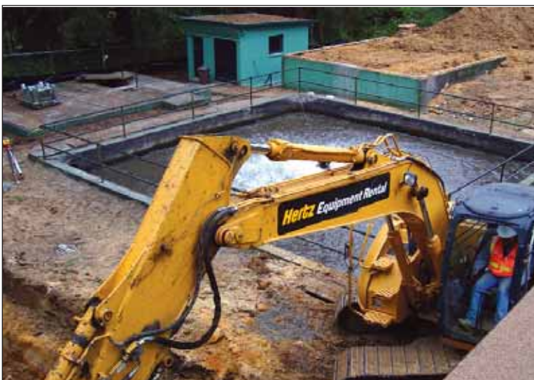
Installation of treatment system
