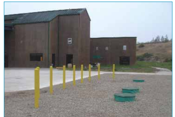
The completed tank installation adjacent to the concrete pad
