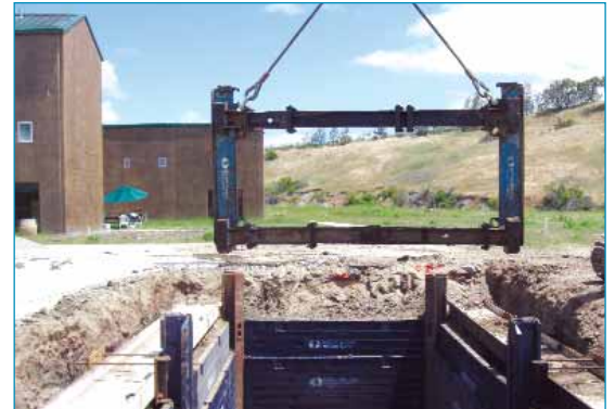
Installing slide rail shoring prior to setting the tank
