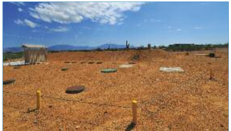
The tank area backfilled with the treatment system installation complete
