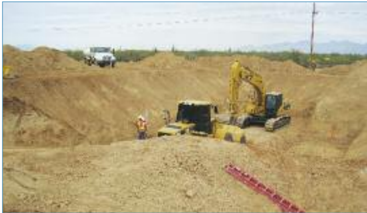
IWS excavates in preparation for setting treatment tanks
