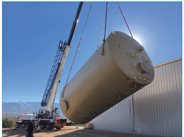
45,000 gallon effluent storage tank being set
