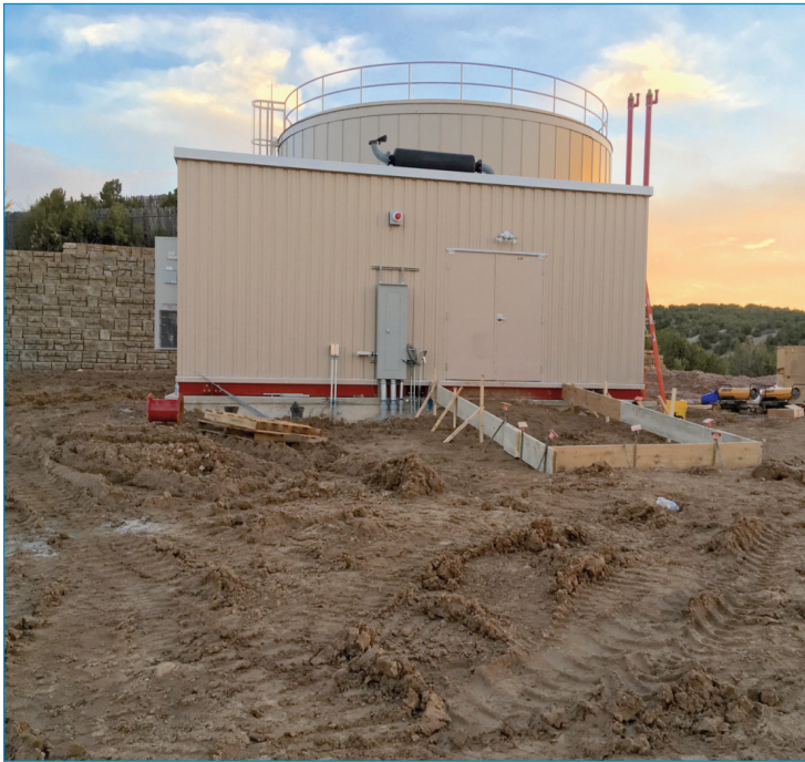
200,000 gallon water storage tank and pump building
