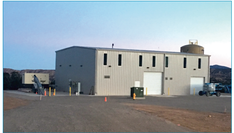
Constructed Metal Treatment Building
