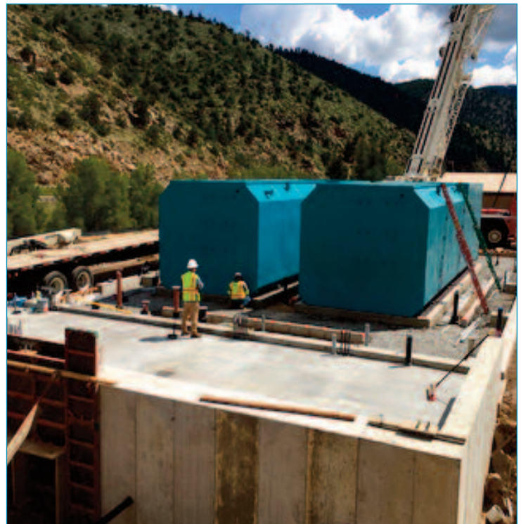
Setting MBR Units on concrete pad
