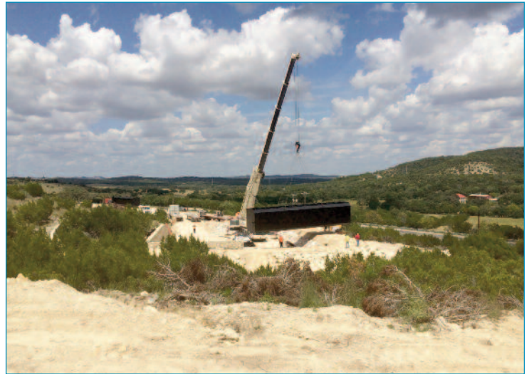
Setting treatment tank with crane
