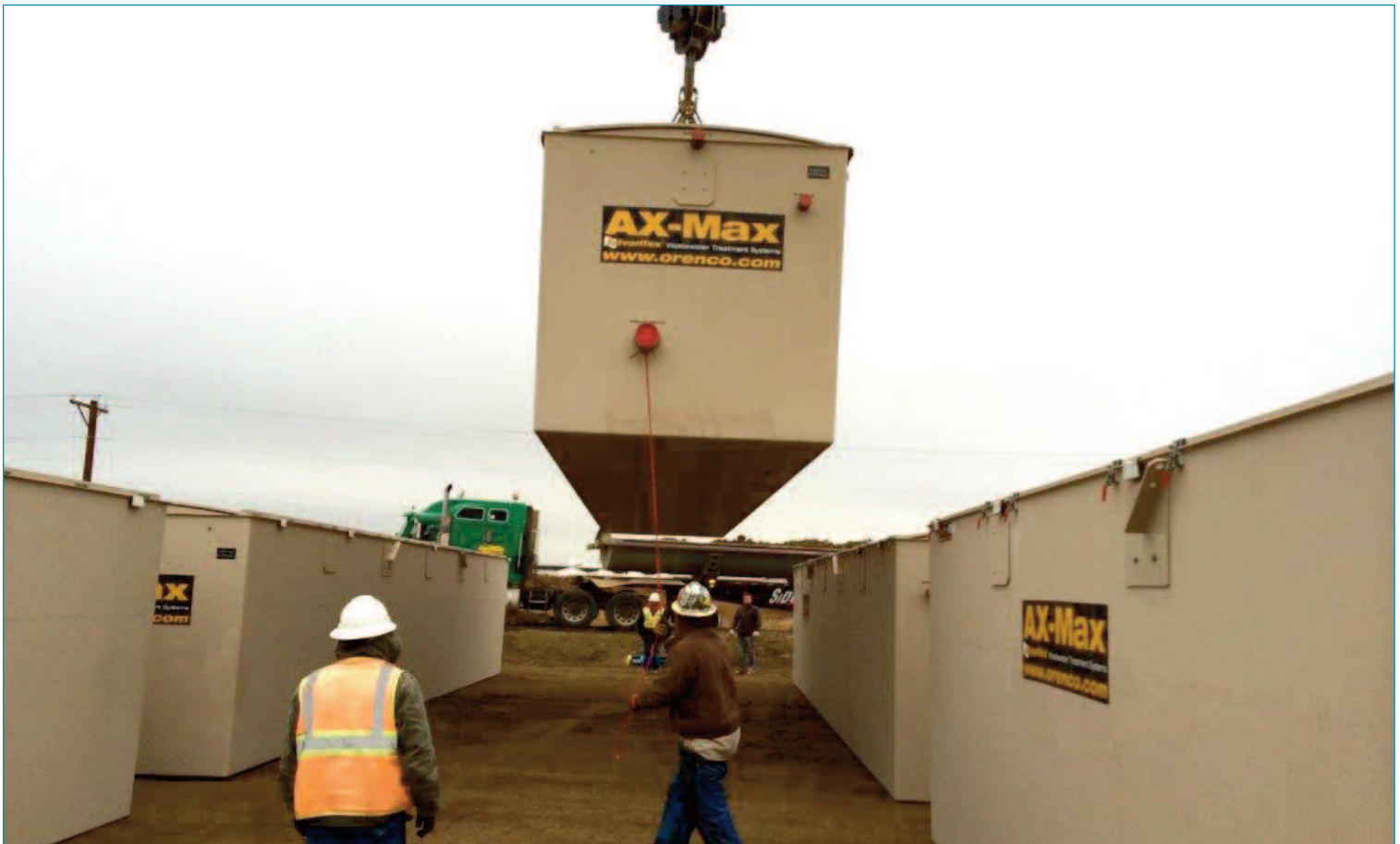
Setting an AX-Max module in position
