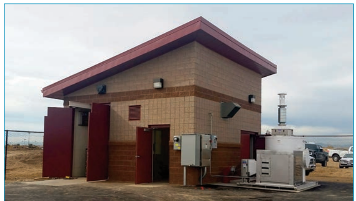
Completed Lift Station
