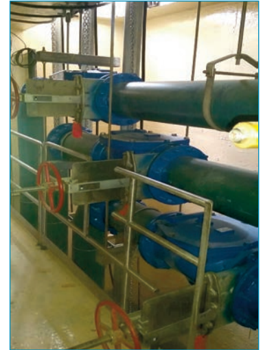
Interior of building
