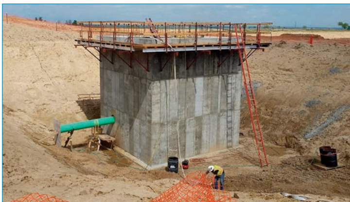
Wet Well Prior to Backfill
