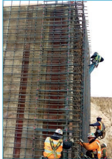
Installing Forms for Wet Well Walls
