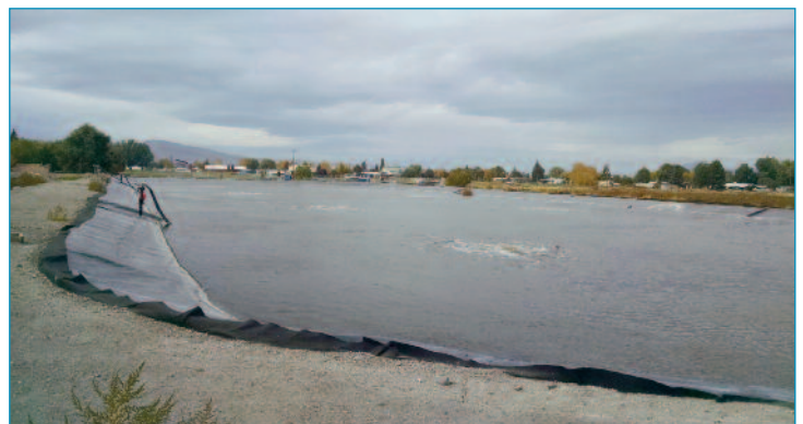
New Aeration Pond
