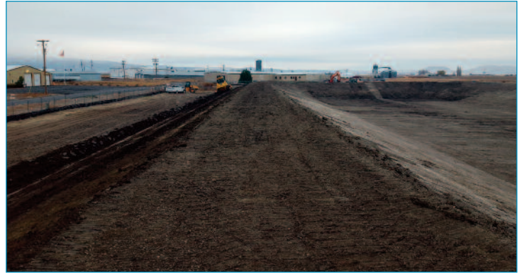
Completing Lagoon Earth Work
