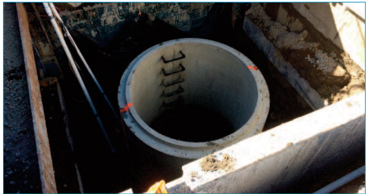
Setting Manhole in Shored Excavation
