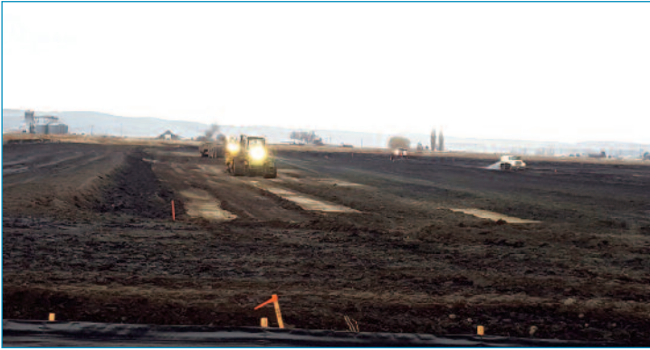
Constructing Effluent Storage Ponds
