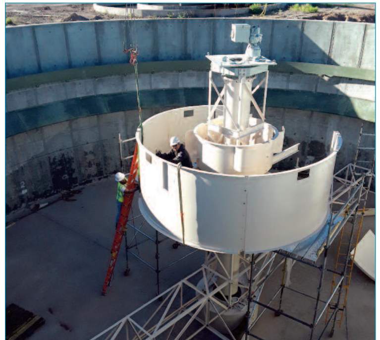
Assembling Clarifier Components
