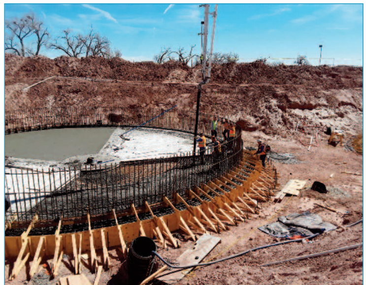
Pouring base of 60 ft diameter clarifier
