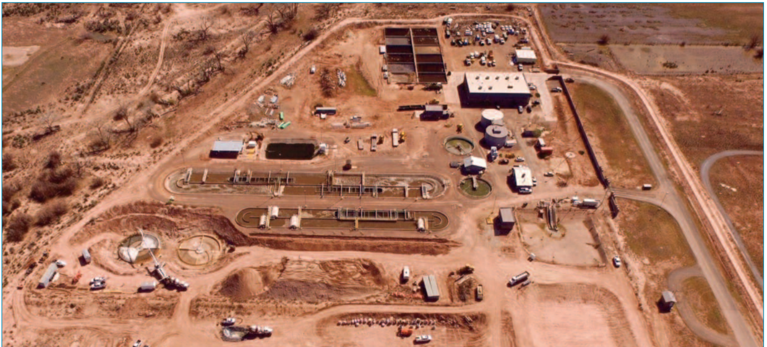
Aerial view of site
