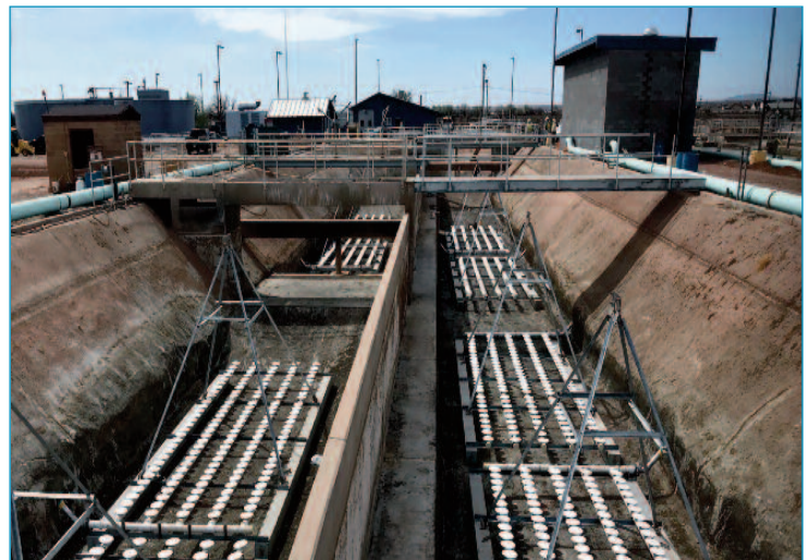
Fine Bubble Diffuser Grid for Oxidation Ditches
