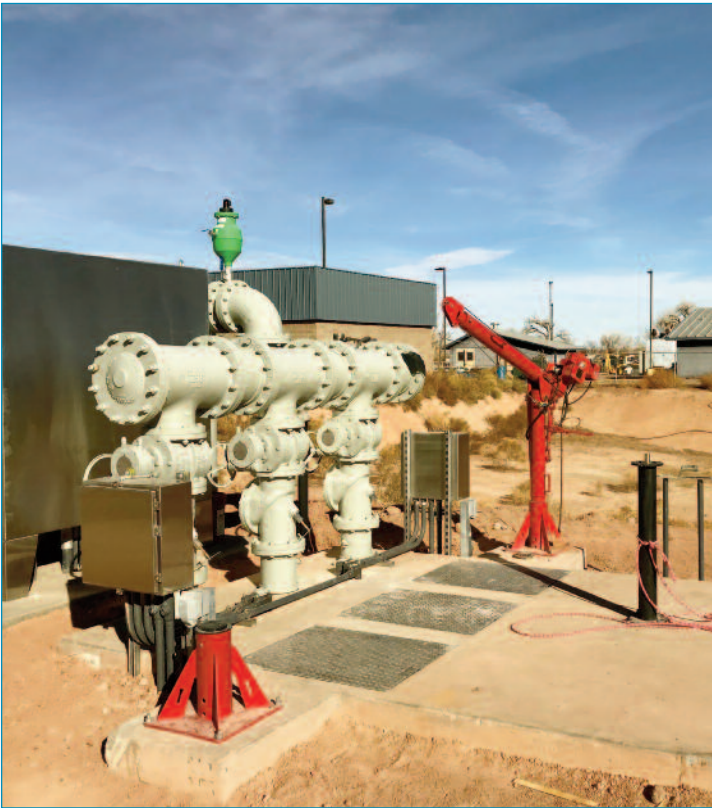
Completed Lift Station
