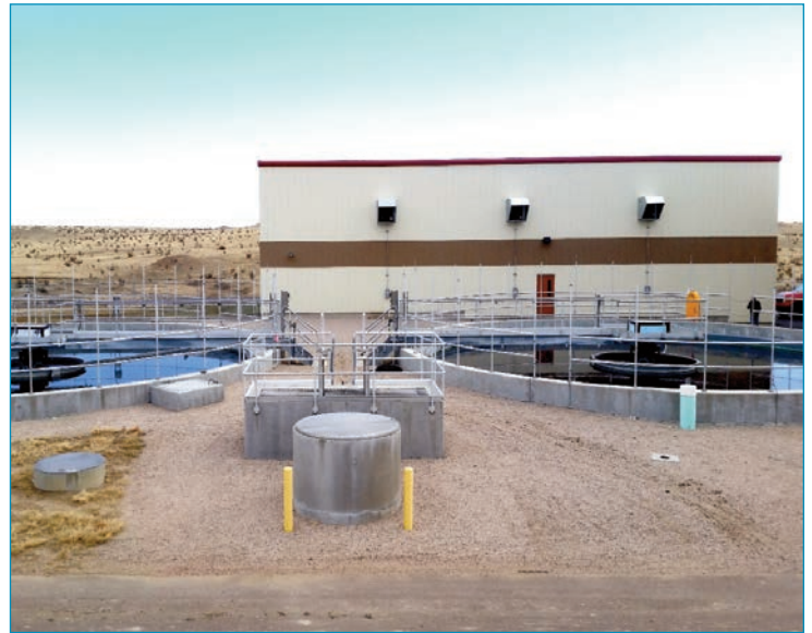
Constructed Metal Treatment Building in the Background
