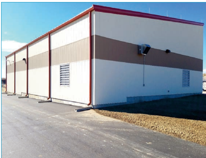
Completed Treatment Building
