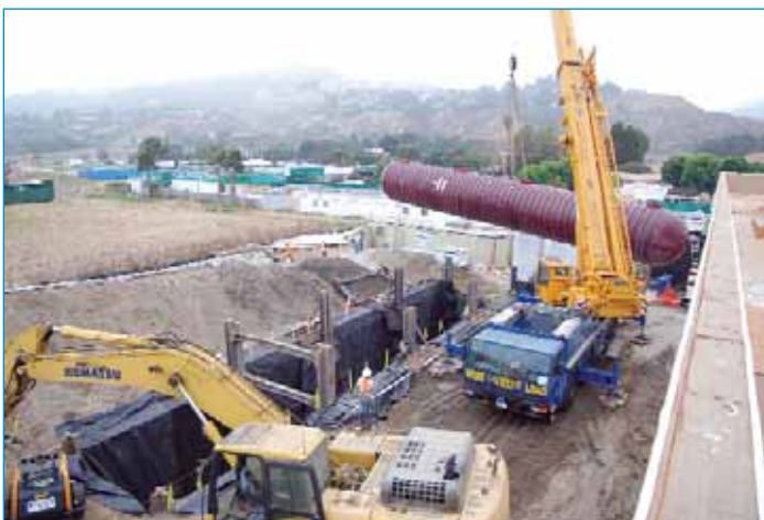
Installation of 75 foot MBR Treatment Tank through shoring structure
