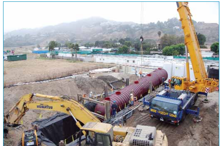
Installation of 75 foot MBR Treatment Tank through shoring structure
