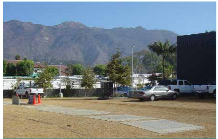
Covers on MBR vaults in the parking lot
