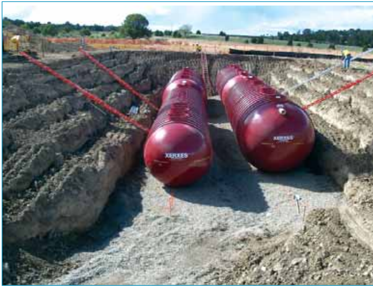
Fiberglass treatment tanks set in excavation
