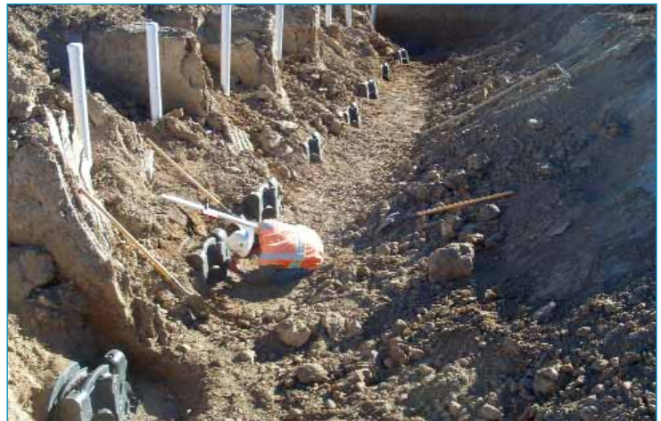
Infiltrator chambers installed for effluent dispersal
