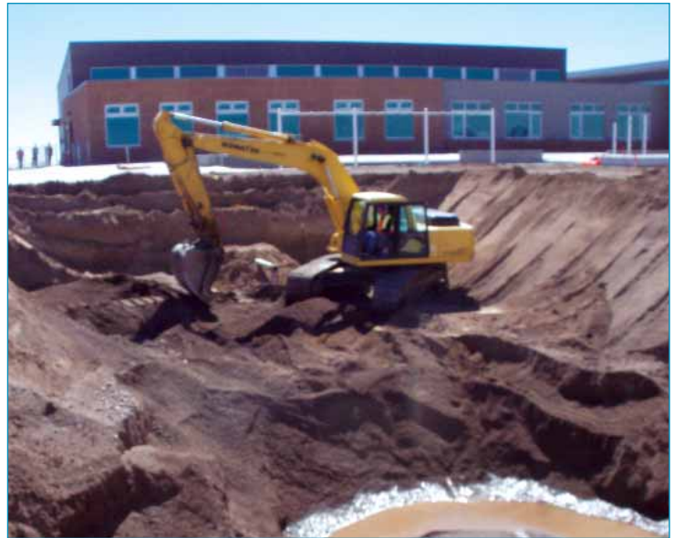
The tank excavation area before the installation
