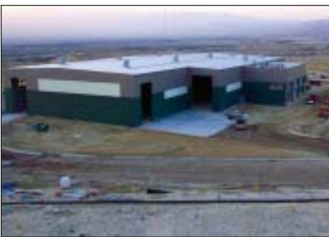
Waste Management Edom Hill Facility
