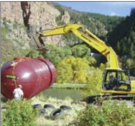
Setting 12,000 gallon septic tank at Hanging Lake
