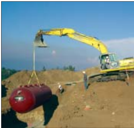
Setting 15,000 Gallon Tank at Ramona Site
