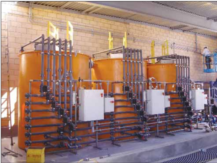
UniPure Brine processing unit (BPU)
